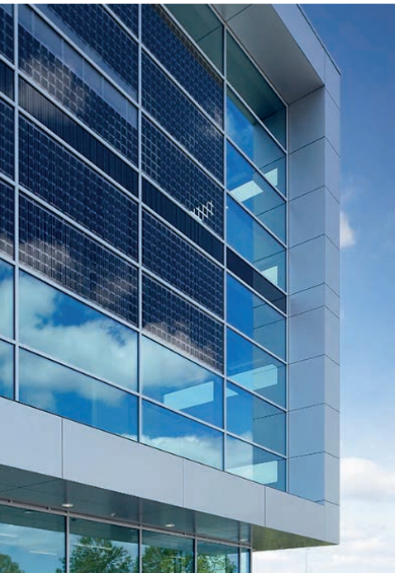
The photovoltaic system of the Brand Experience Center is approx. 450 m 2 and supplies around 42,000 kilowatt hours of electricity per year. (Those: AUDI AG)
